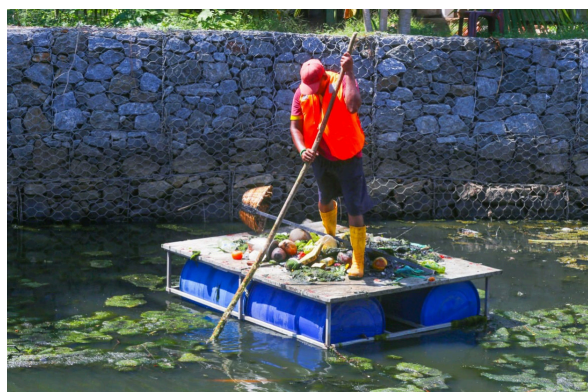
Waste Retainer installed across the Abru stream and removing the waste retained on that retainer
